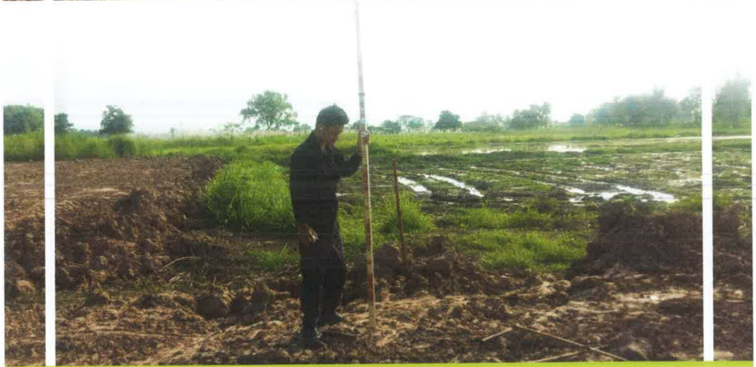
Survey design clearing on site
